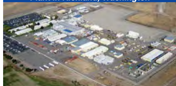
Figure 7-1. AREVA Nuclear Fuel Services Plant in Richland, Washington
