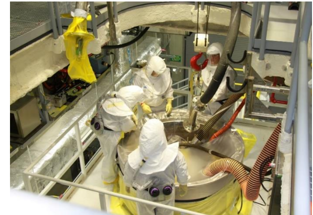
K West Reactor Basin sludge retrieval
