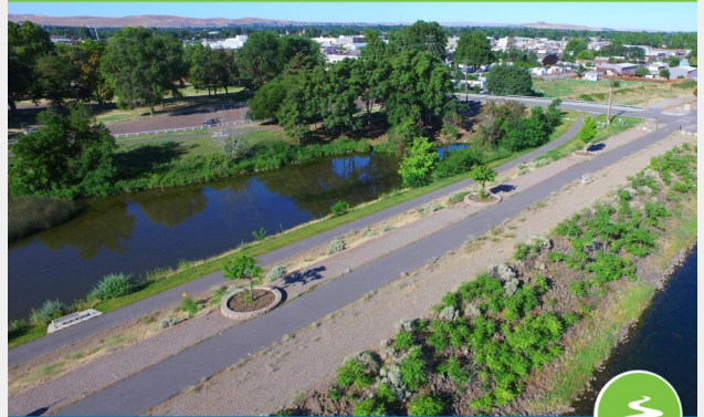
LEVEE AT CLOVER ISLAND
