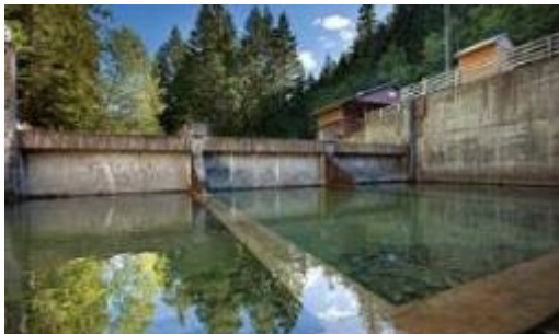
Packwood Lake Hydroelectric Project (27 MWe)
