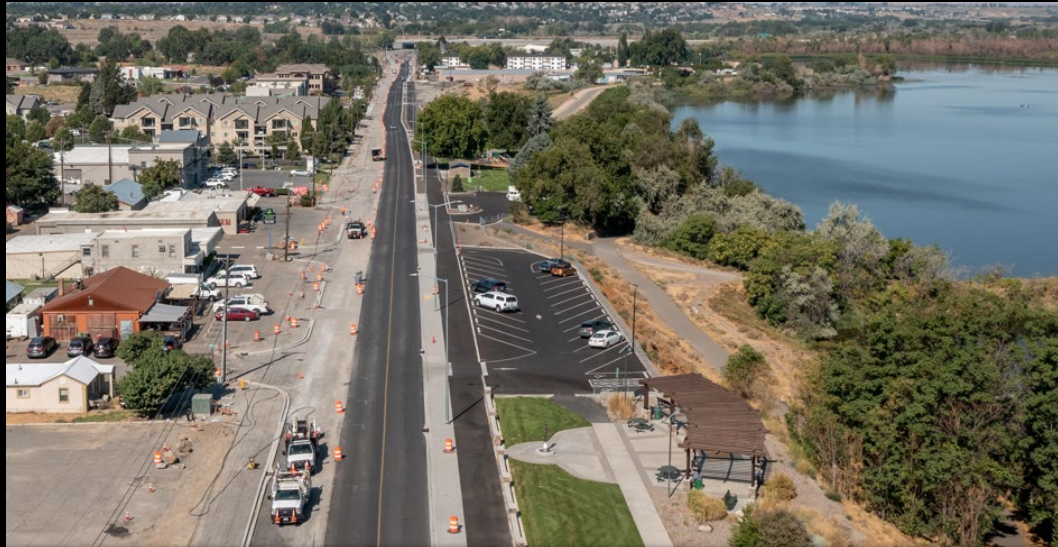
Supported City of Richland in transforming their Island View neighborhood and undergrounding of utilities
