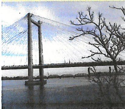
Below: Cable Bridge (foreground) and Burlington Northern Santa Fe railroad bridge
